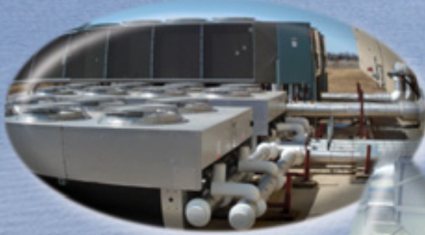
Above, dry coolers, chillers and interconnecting piping flow into Albany International's Kaukauna facility. Right, a duct drop descends from a large roof-mounted air-handling unit. Far right, boilers and pumps are part of a high-efficiency boiler system installed by Bassett.
